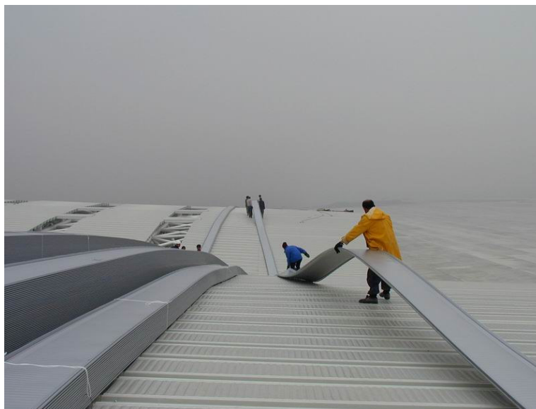
The sheets as long as the roof pitch
